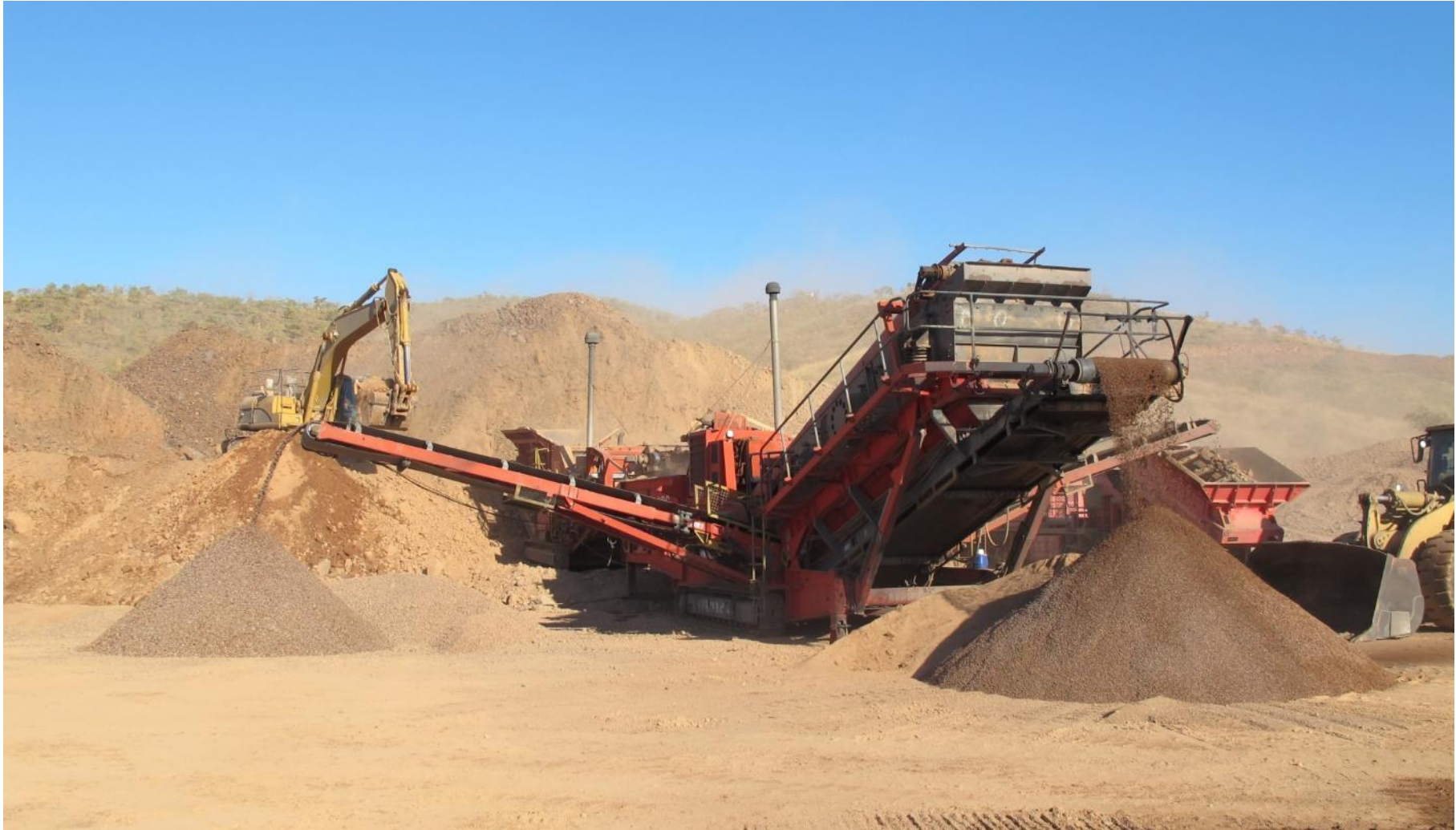
Bentonite Laydown & Cover Material Crushing Plant
