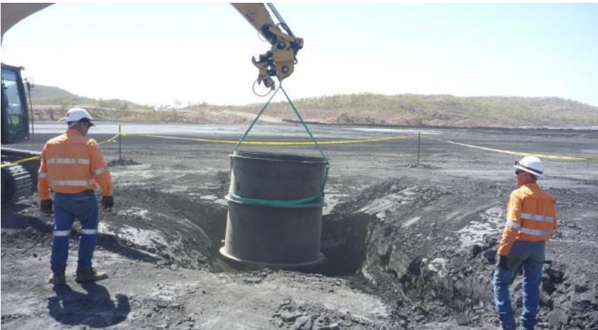
Lysimeter Placement Below Tailings Beach
