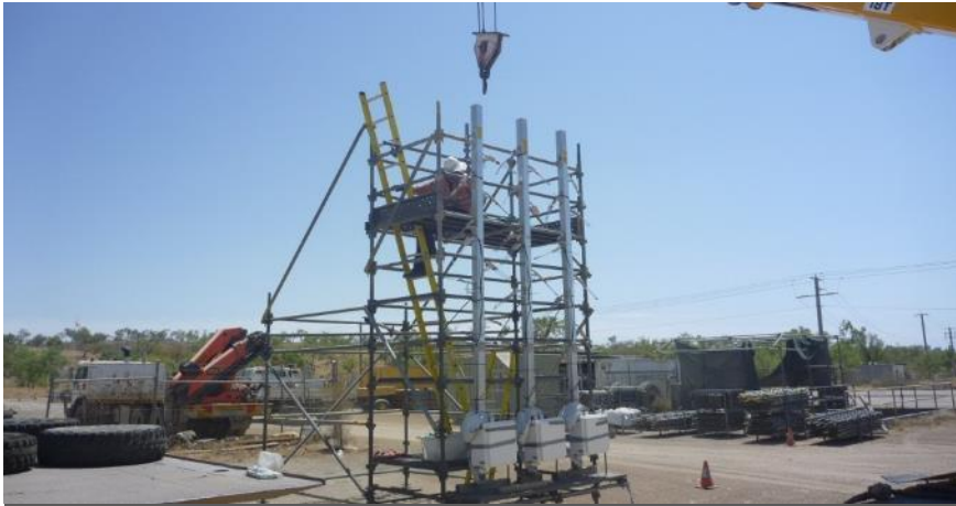
Instrumentation Tree Pre-wiring
