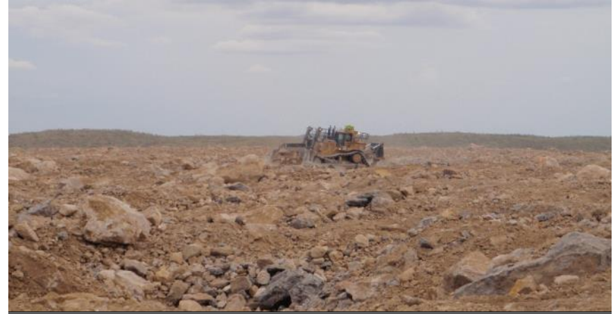
8. Muting of Storage Layer Using D11 Dozer
