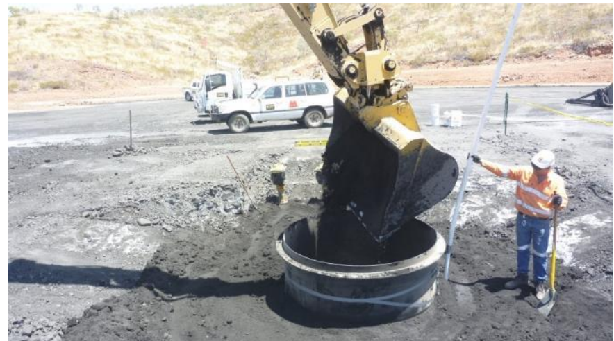
Backfill Lysimeter with Tailings
