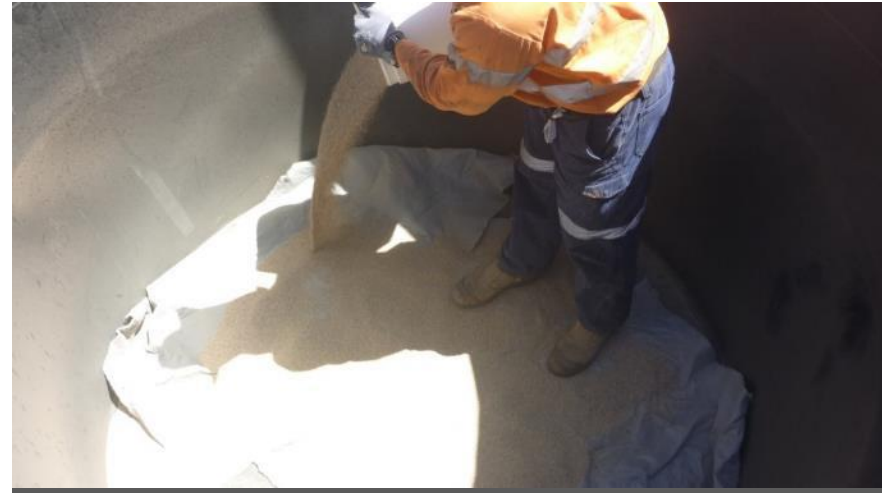
Backfill Lysimeter with Filter Sand
