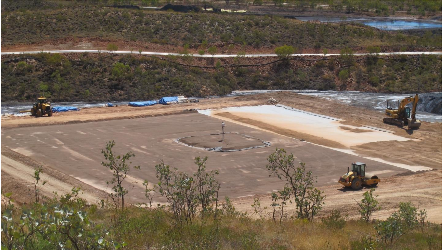
Laying of Geosynthetic Clay Liner
