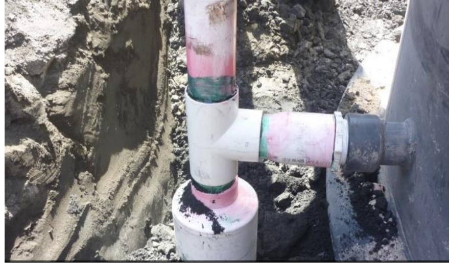
Lysimeter Sump Installation
