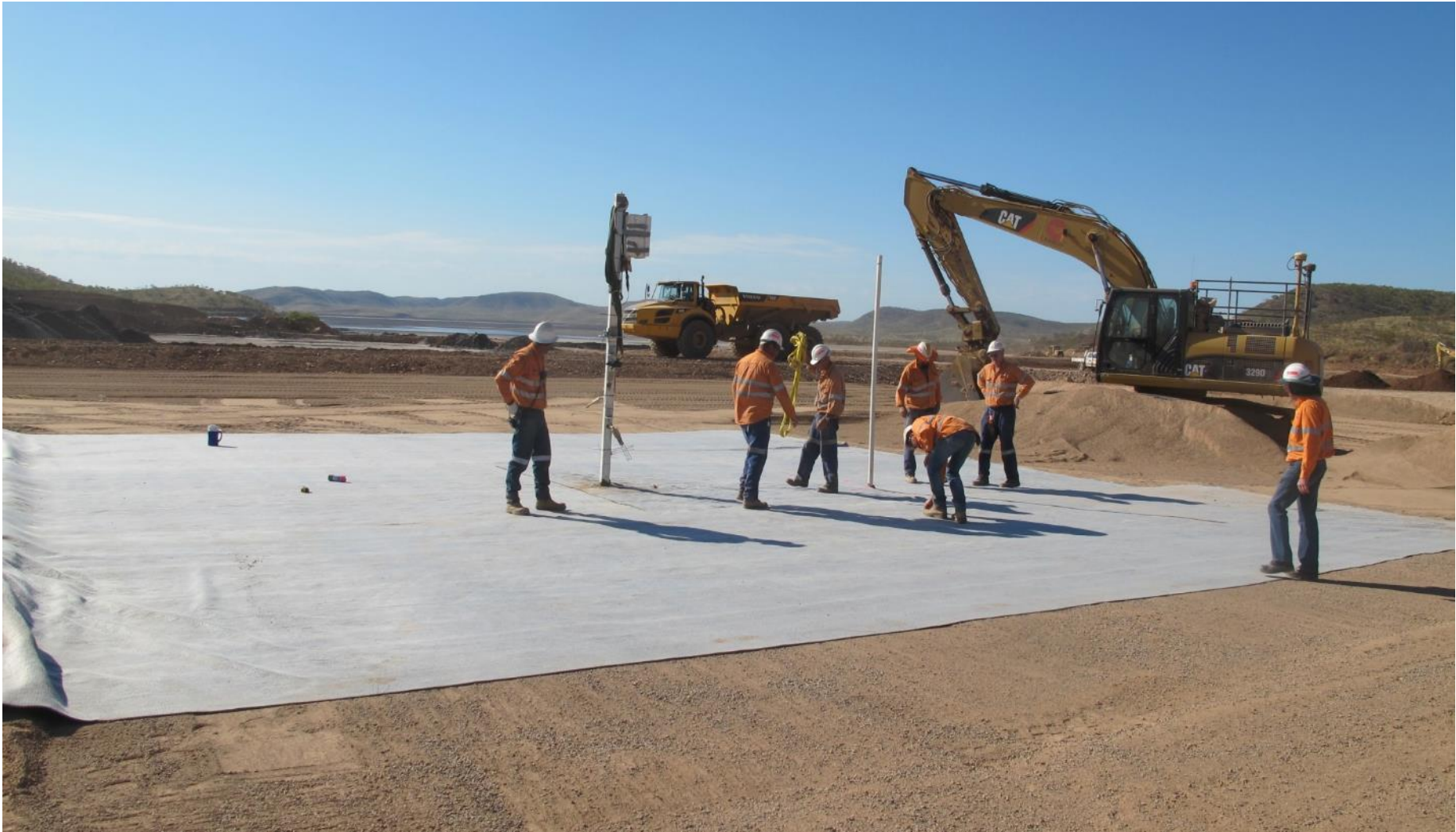
Laying of Geosynthetic Clay Liner
