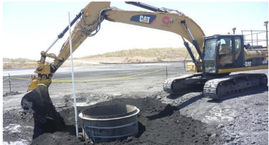
Backfill Around Lysimeter and Sump
