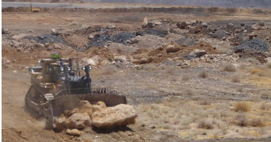
1. Removal of Oversized Material
