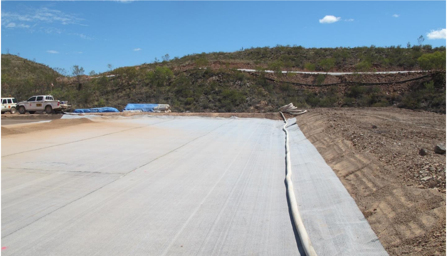
Laying of Geosynthetic Clay Liner
