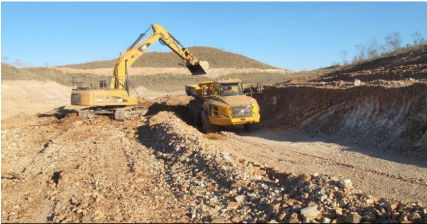
Embankment Clay Material Excavated from Borrow
