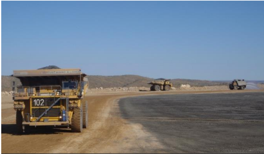
5. RPL Compaction with Fully Laden 830E
