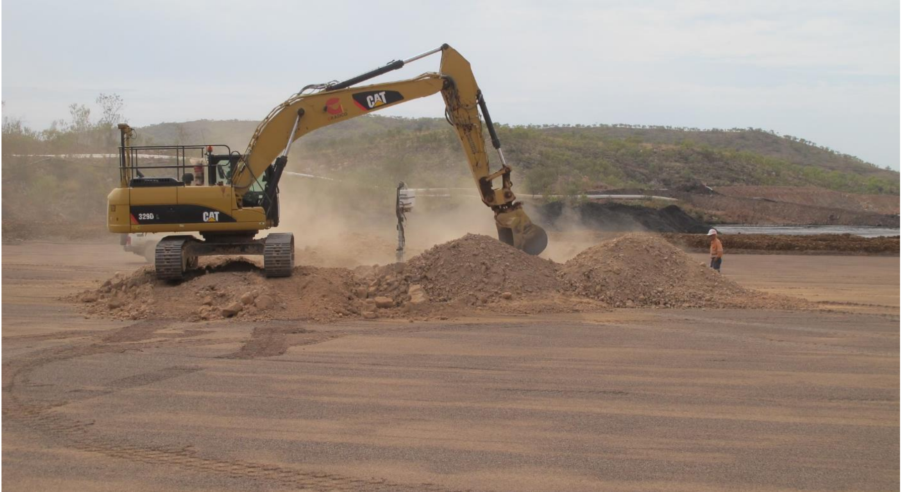
Placement of Rock Mulch Layer Around Instrument Tree
