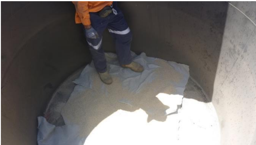
Geo-fabric Filter Placed on Base of Lysimeter
