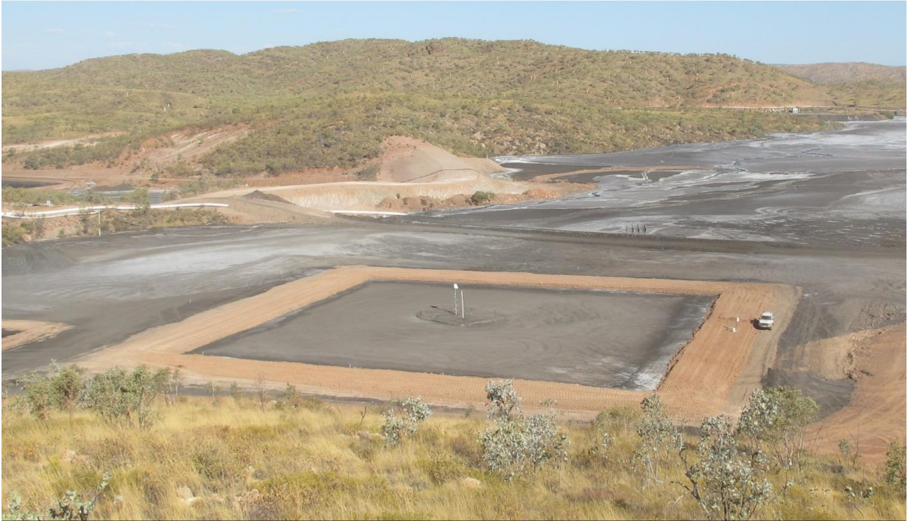
Cover Trial Cell Embankment Foundation & Instrumentation Installed Centrally
