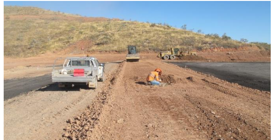
Embankment Compaction Testing
