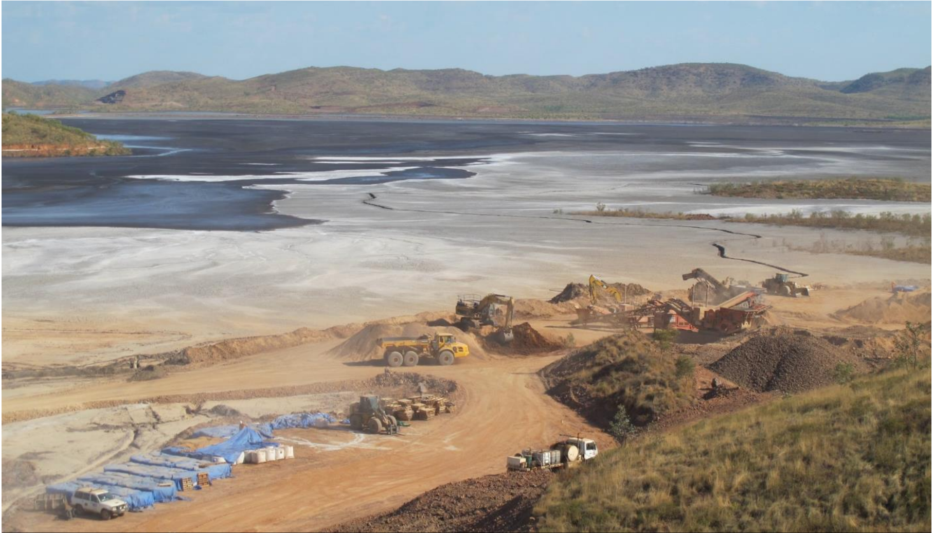
Bentonite Laydown & Cover Material Crushing Plant
