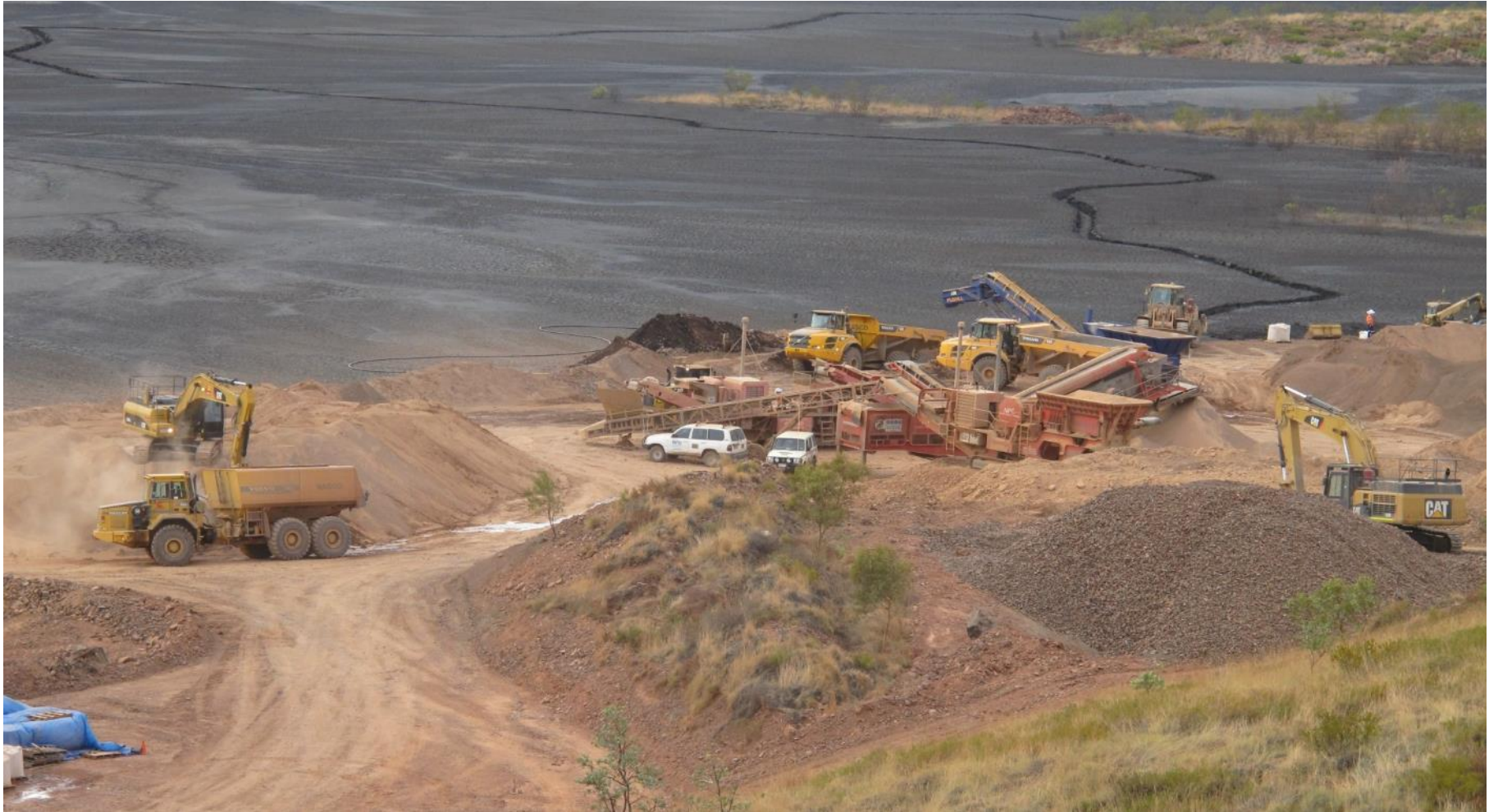
Bentonite Laydown & Cover Material Crushing Plant
