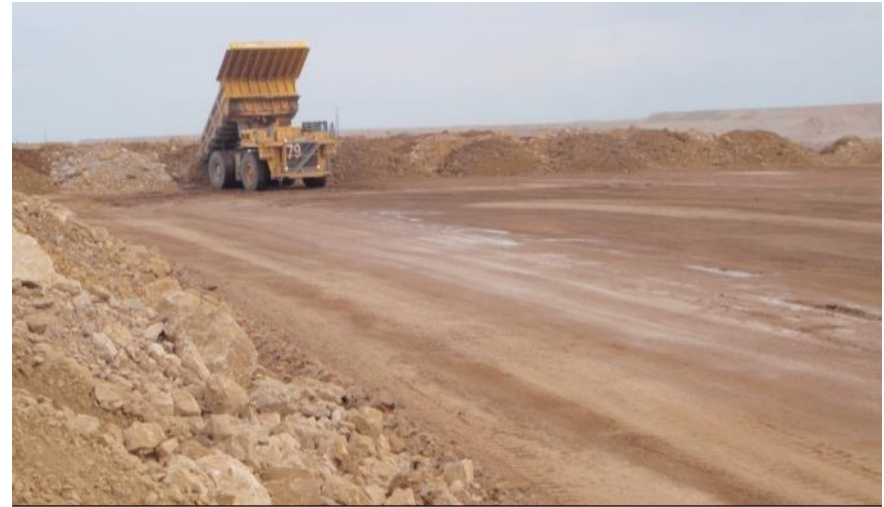
7. Dolomite Storage Layer Paddock Dumped Out
