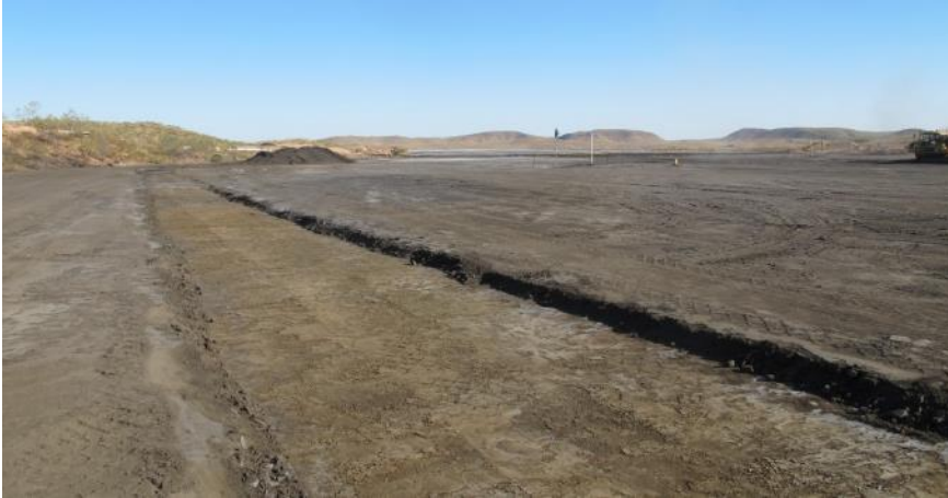
Embankment Keyed Into Tailings Beach
