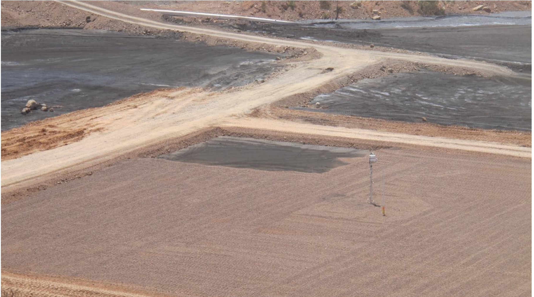
Placement of Capillary Break Material
