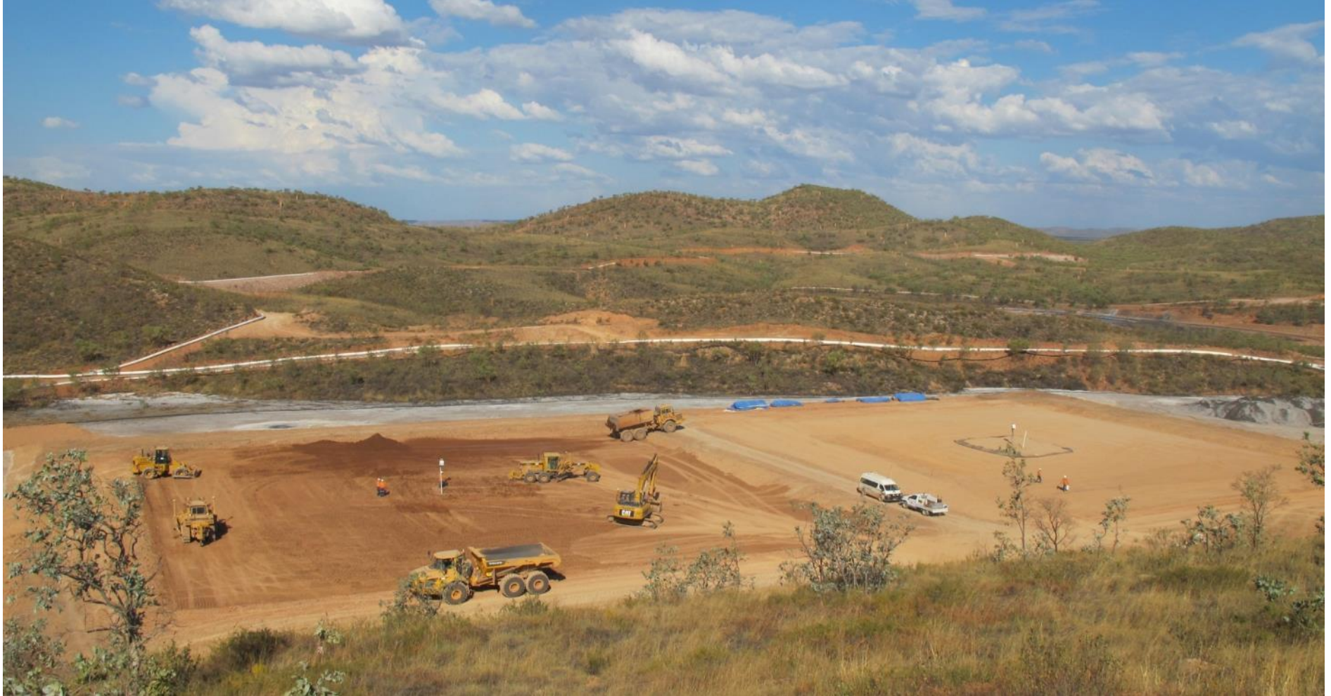
Placement and Compaction of RPL
