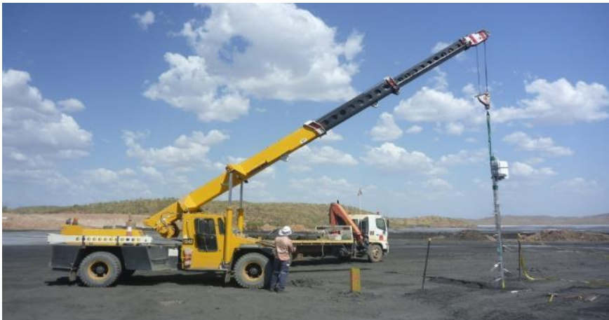
Instrumentation Tree Placement
