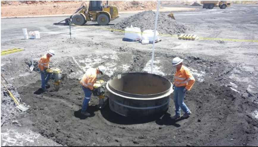
Compaction of Backfilled Tailings
