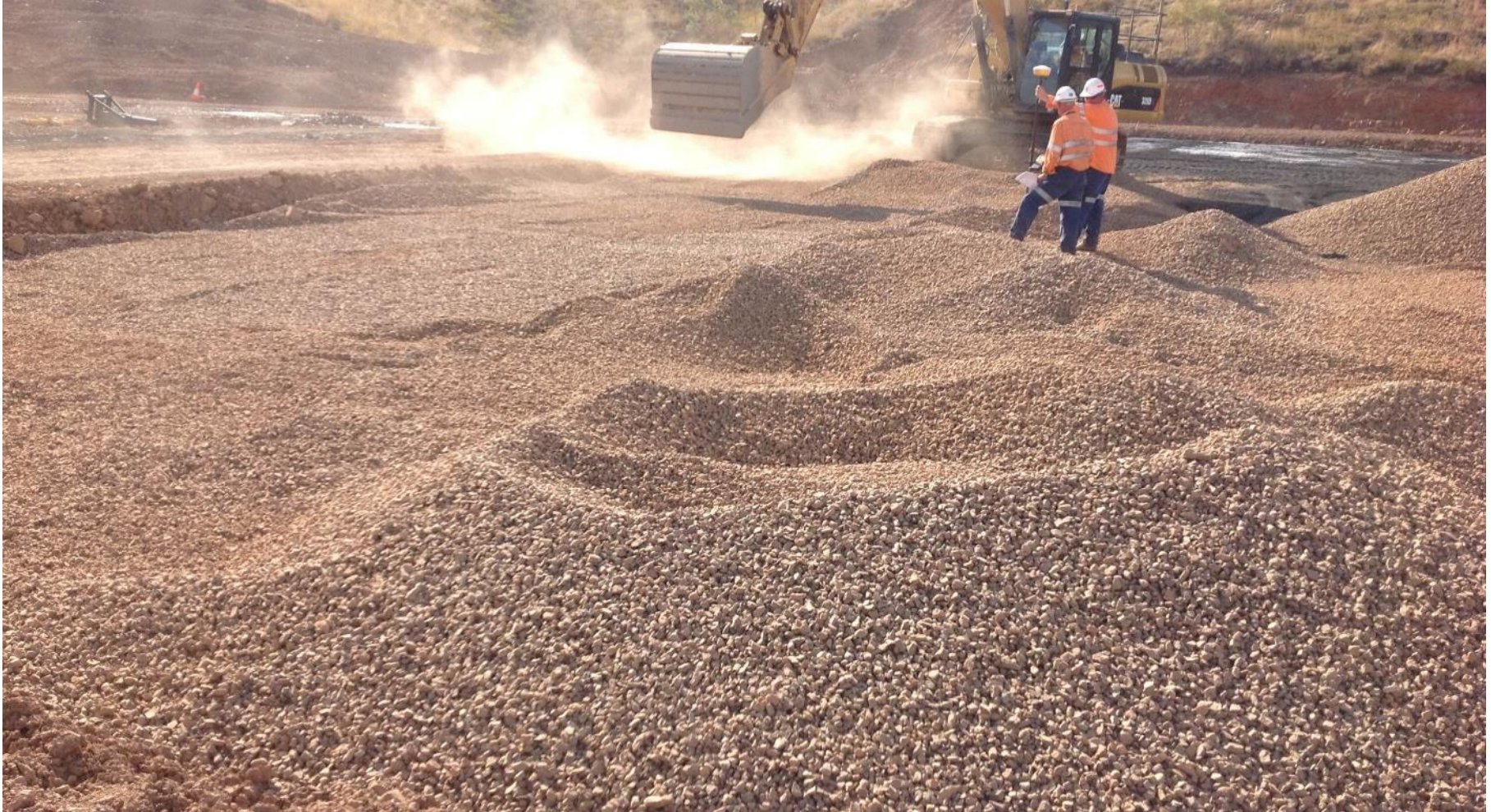
Placement of Capillary Break Material
