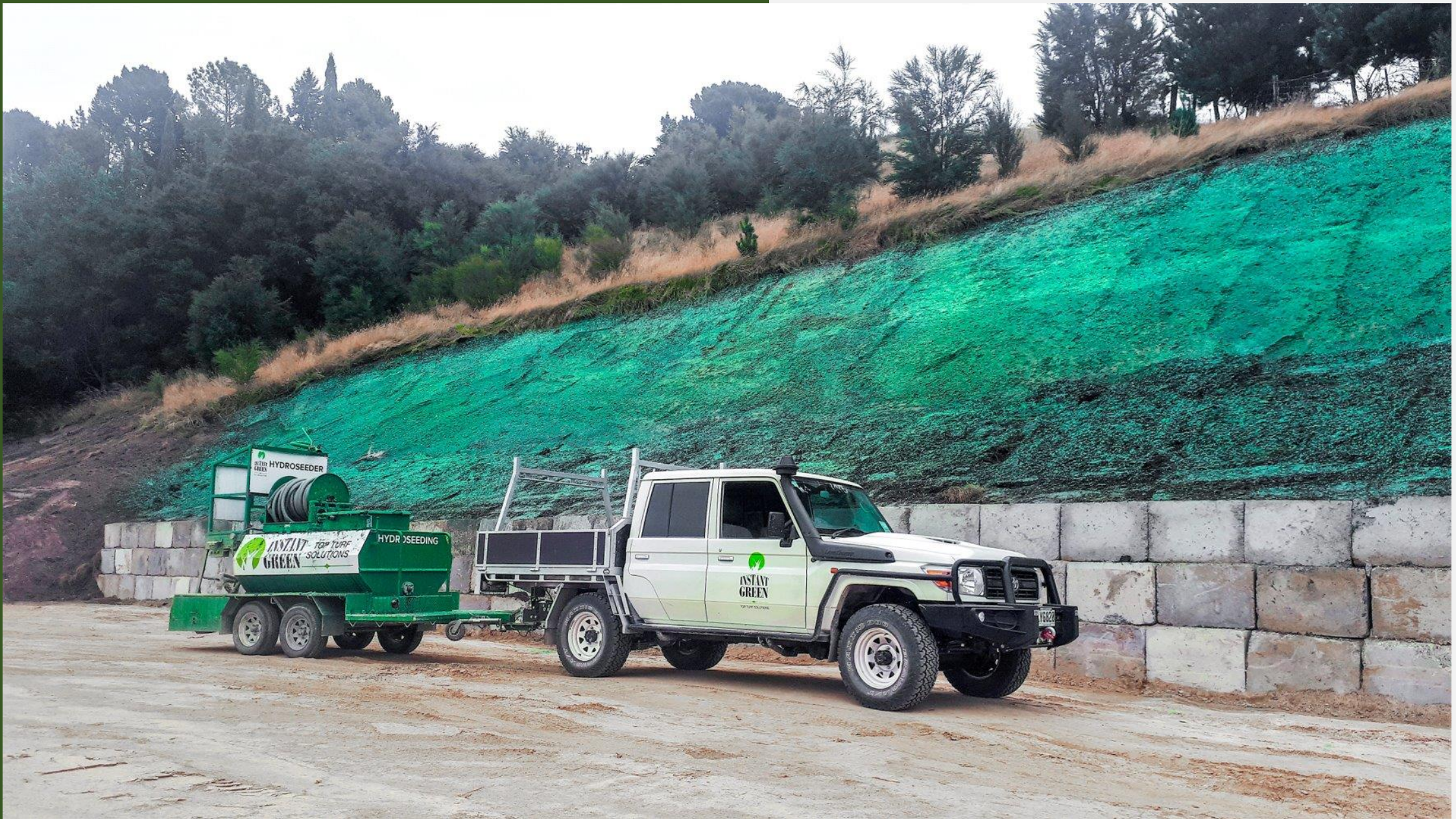
2007: LAND CRUISER + TRAILER COMPLETING SMALL PROJECTS
