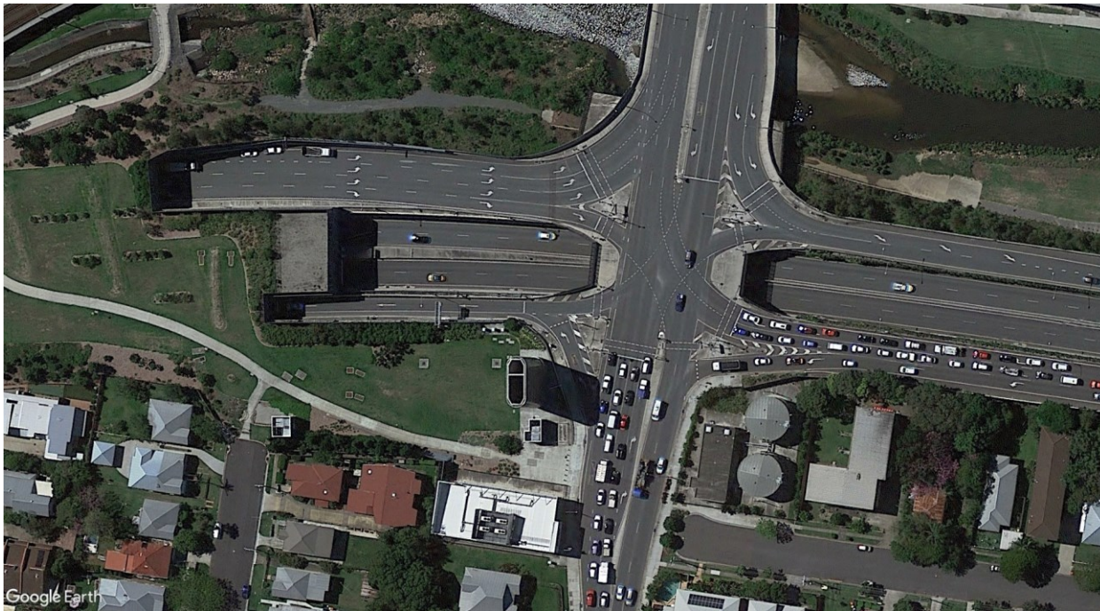
Brisbane Airport Tunnel Portals and Interchange
