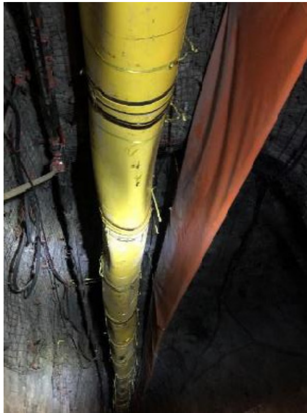
FIG 2 – 762 mm thermoplastic ducting installation showing buckling.
