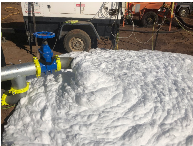
FIG 2 – Photograph of N 2 foam from a pipeline feed showing stand-up capability.
