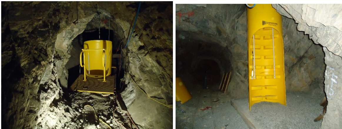
FIG 2 – Safescape Laddertube installed at Colorado School of Mines Edgar Mine.
