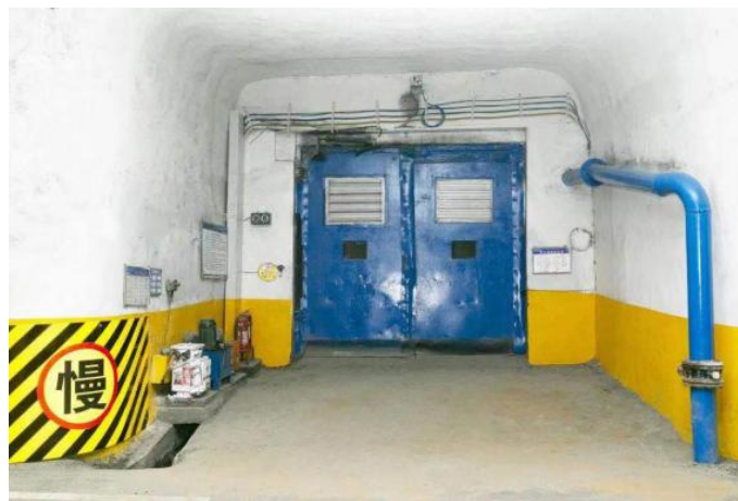
FIG 13 – Automatic damper of Yubei Caojiatan Mining Company.
