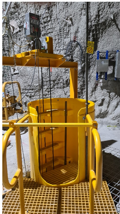
FIG 8 – Tractelift system installed in Safescape Laddertube.
