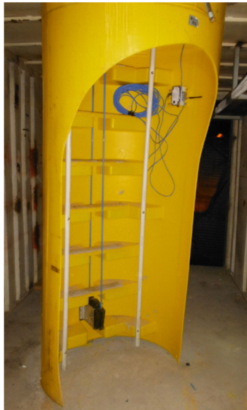
FIG 7 – Extended Ladder Climb Assist with an Easy Climb Controller.
