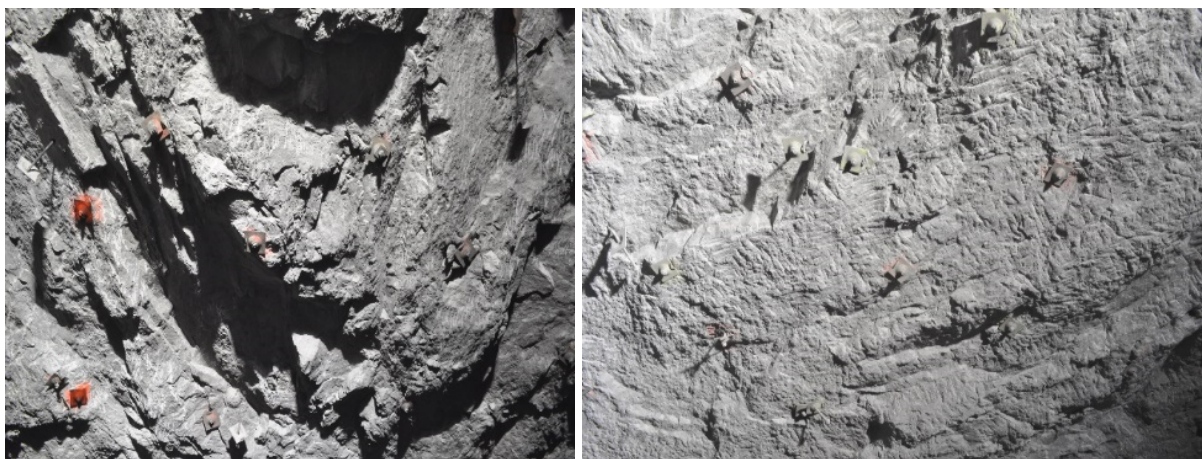
FIG 1 – Images for hazardous (left) and non-hazardous (right) roof conditions.
