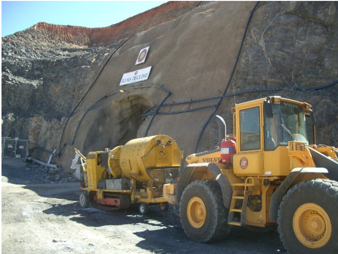
FIG 4 – Mobile vacuum unit towed out form underground nickel mine in WA.
