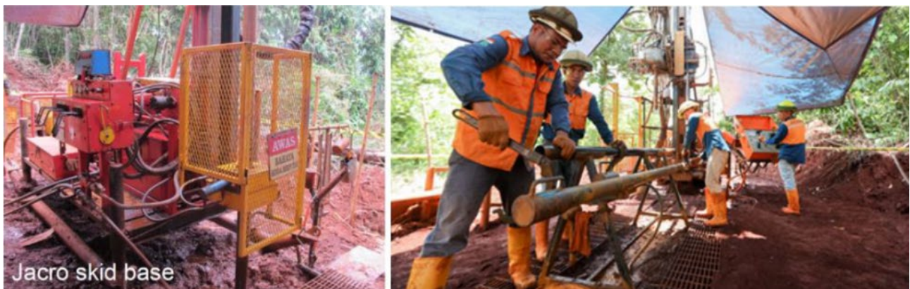
FIG 4 – Drilling and sampling activity using HQ3 core size.
