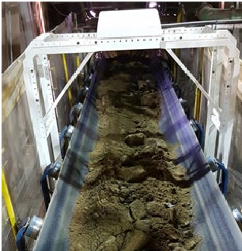
FIG 3 – 3D Infrared camera PSD analyser which measures belt speed and volume and calculates tonnes per hour using a bulk density estimate (source: Scantech International Pty Ltd).
