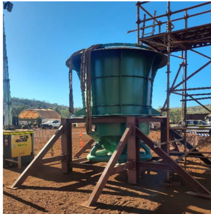
FIG 6 – Rotable Coarse Section at site.
