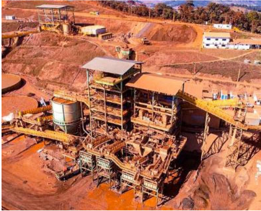
FIG 1 – JMN processing plant.
