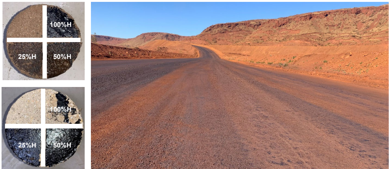
FIG 2 – Examples of capping layer assessment (left), and HaulPac-capped mine haul road.
