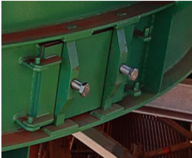
FIG 7 – New inspection hatch.
