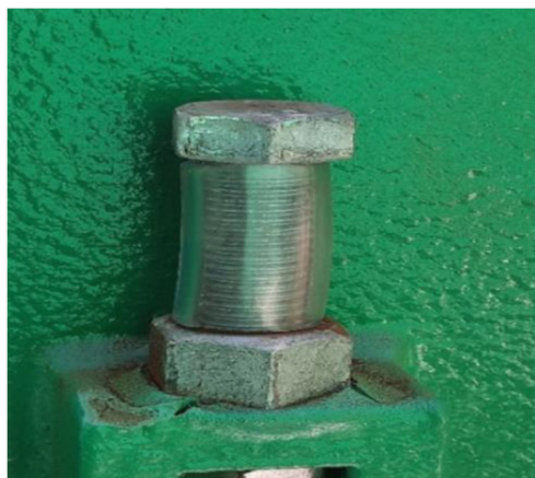
FIG 10 – Plastic sleeve protection.
