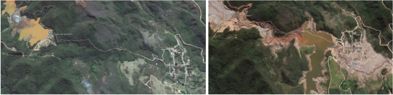
FIG 1 – Aerial view of the dam (before and after the collapse, 2015; Bento Rodriguez village).
