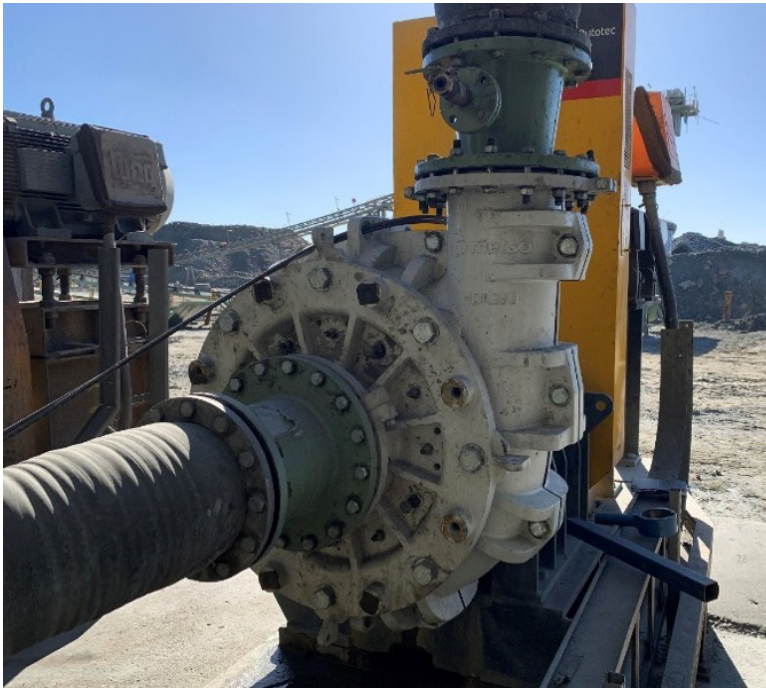
Newly installed MD pump ready for commissioning
