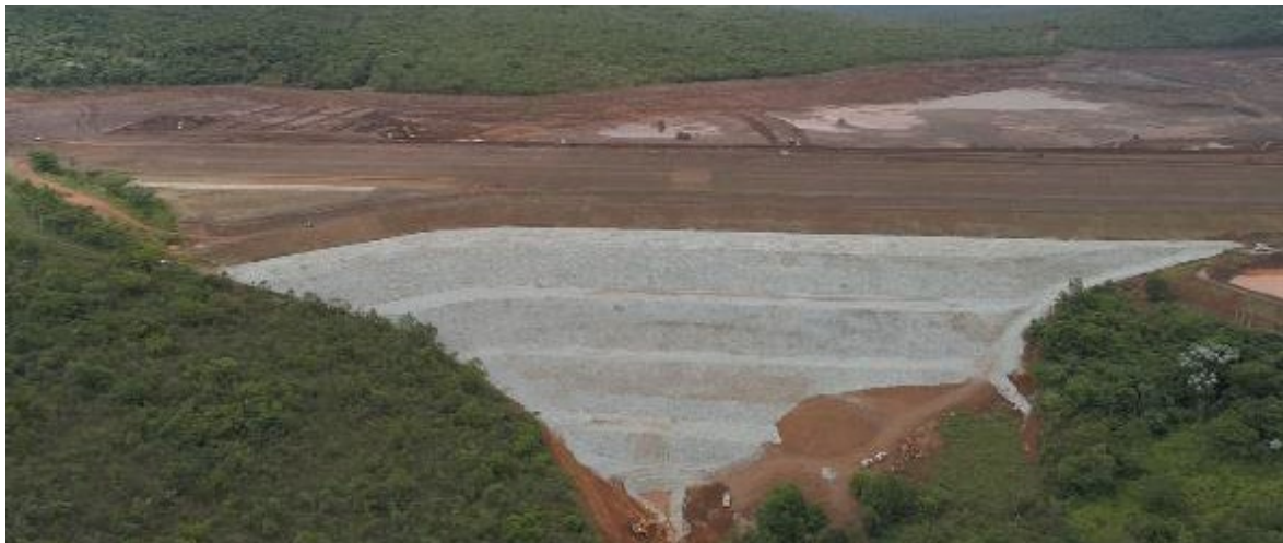
FIG 4 – Downstream reinforcement, November 2019.
