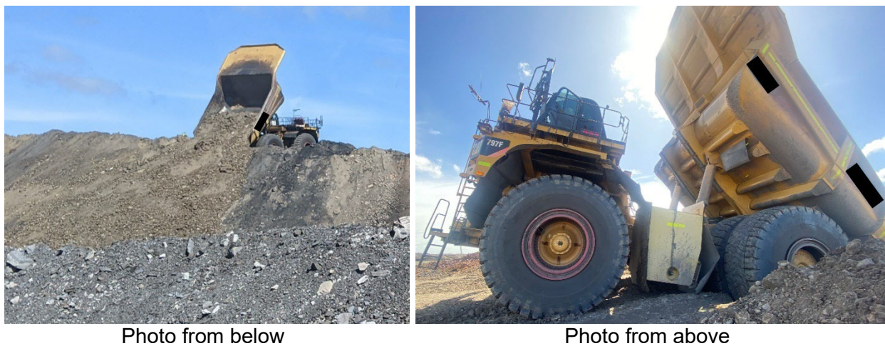
FIG 4 – Photos of failure in 20 m high tip head.
