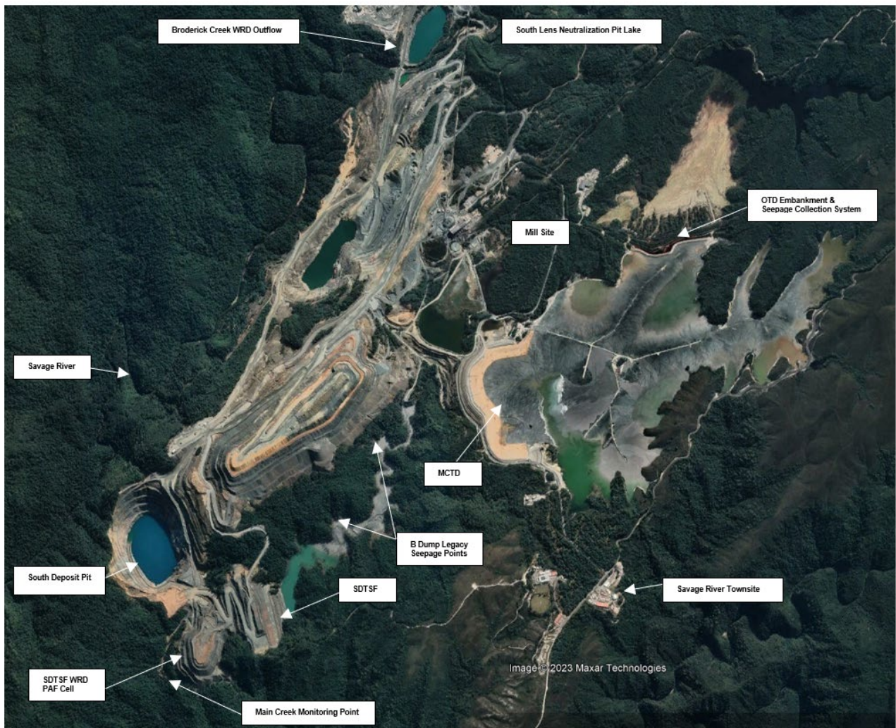
FIG 1 – General arrangement of site (Google Earth 2023).
