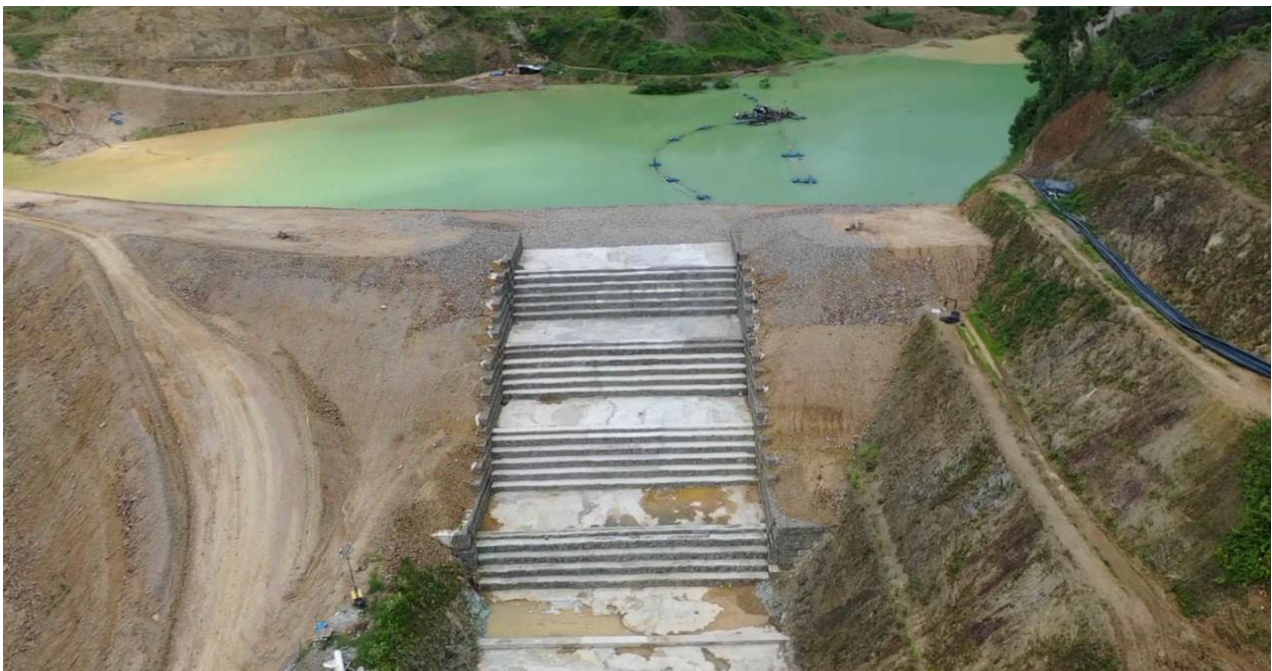
FIG 6 – Completed spillway.
