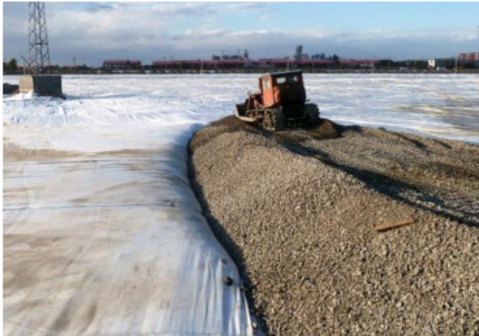
FIG 12 – Finger dyke construction (source: TenCate (2020)).
