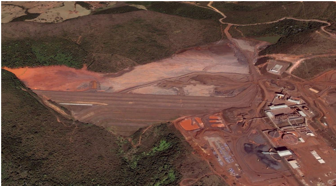
FIG 19 – Aerial view of the area called Central Dam, 2014.
