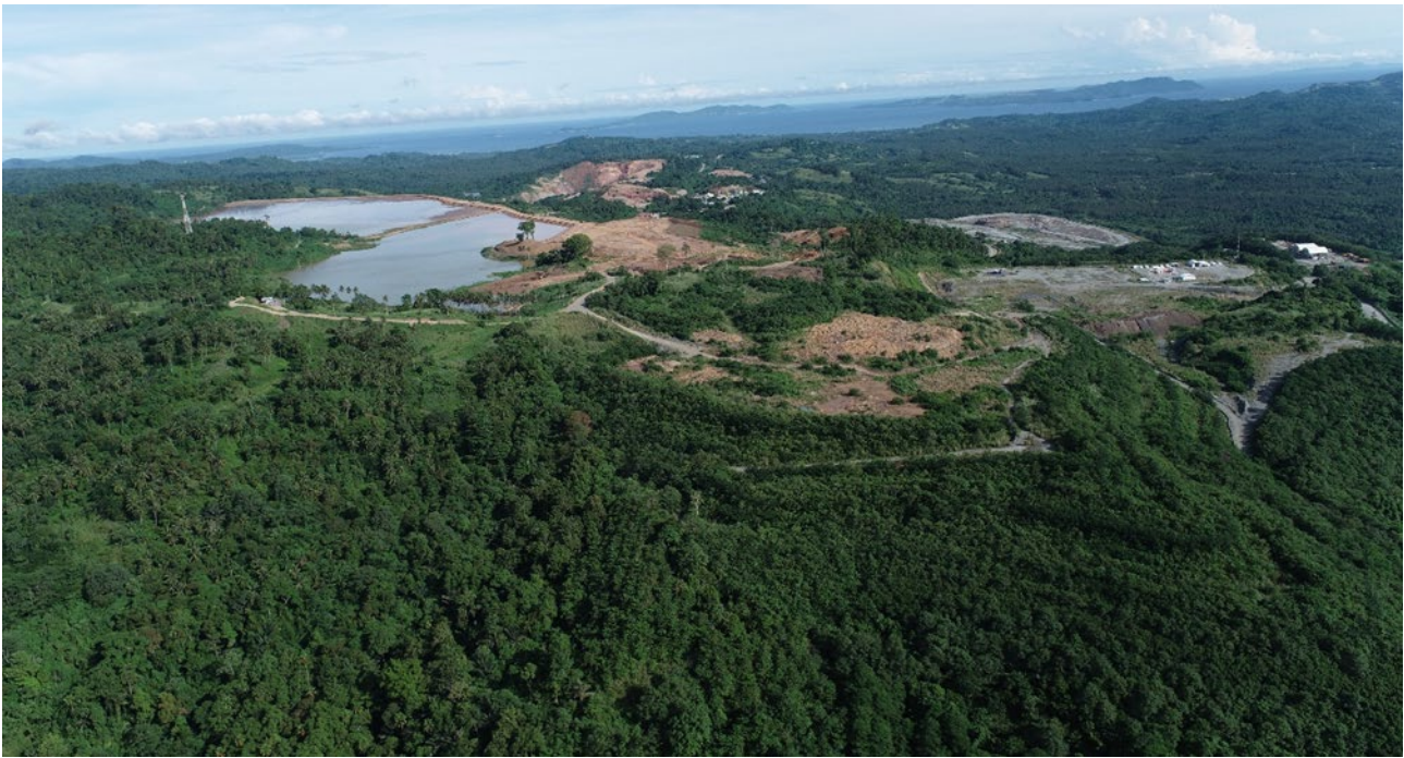
FIG 1 – View of existing TSF with plant site in centre of photo.
