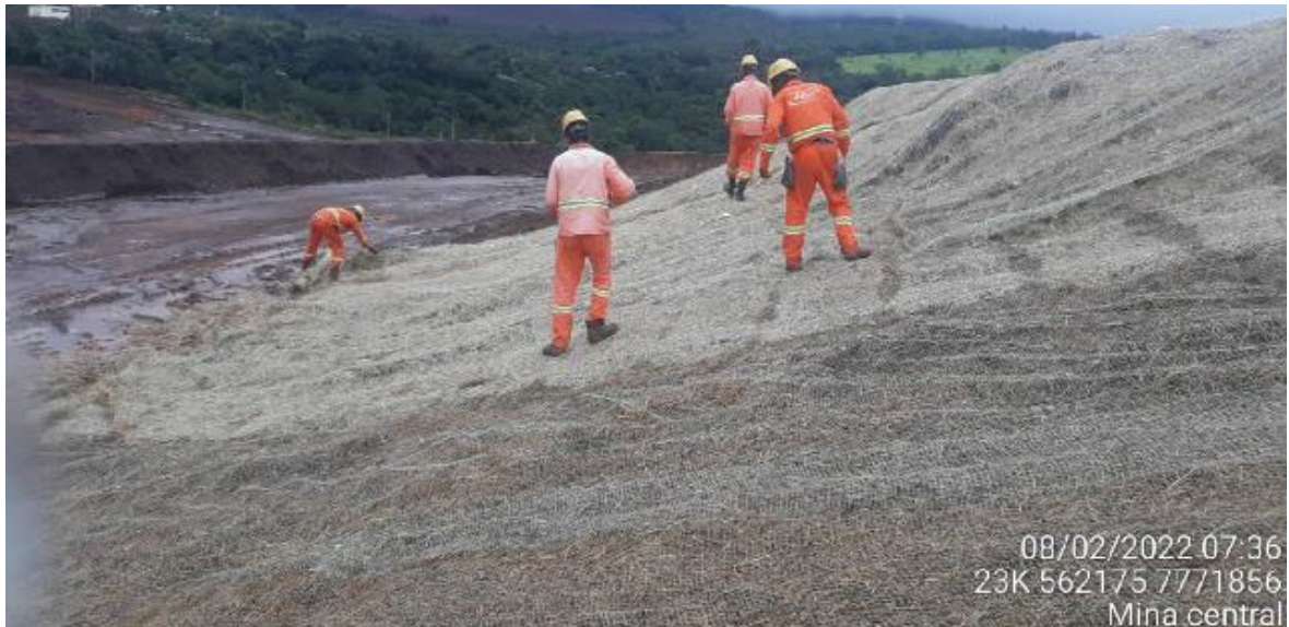
FIG 14 – Anti-erosion bio-blanket.
