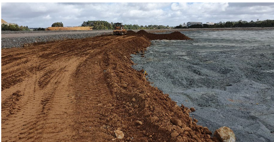
FIG 8 – Clay cover placement.
