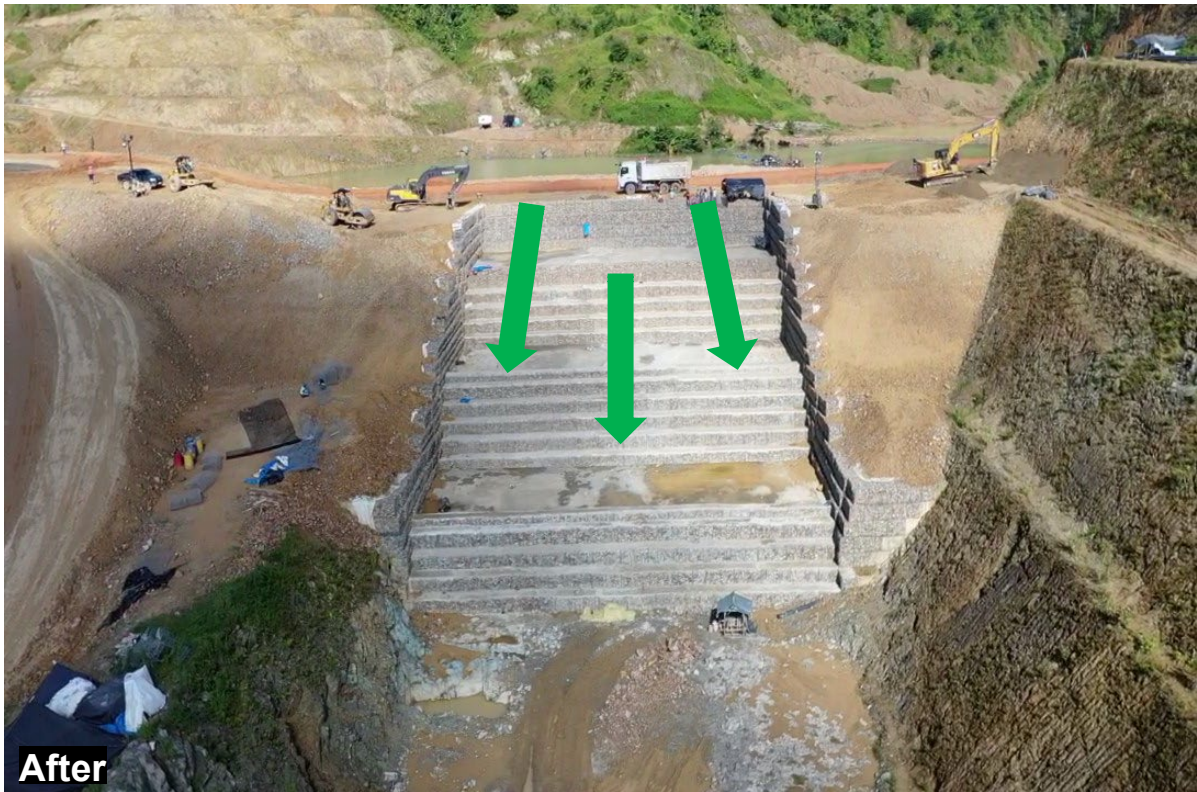
FIG 5 – Properly constructed spillway.
