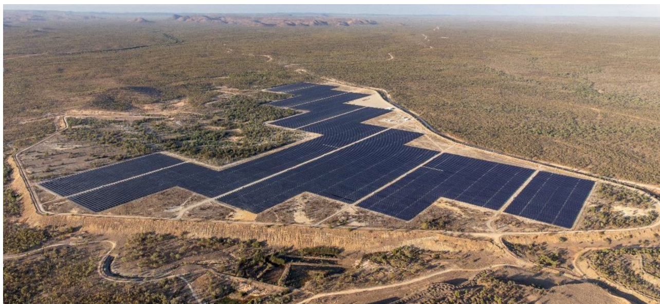
FIG 1 – 50 MW Kidston Solar built on the Kidston tailings dam.
