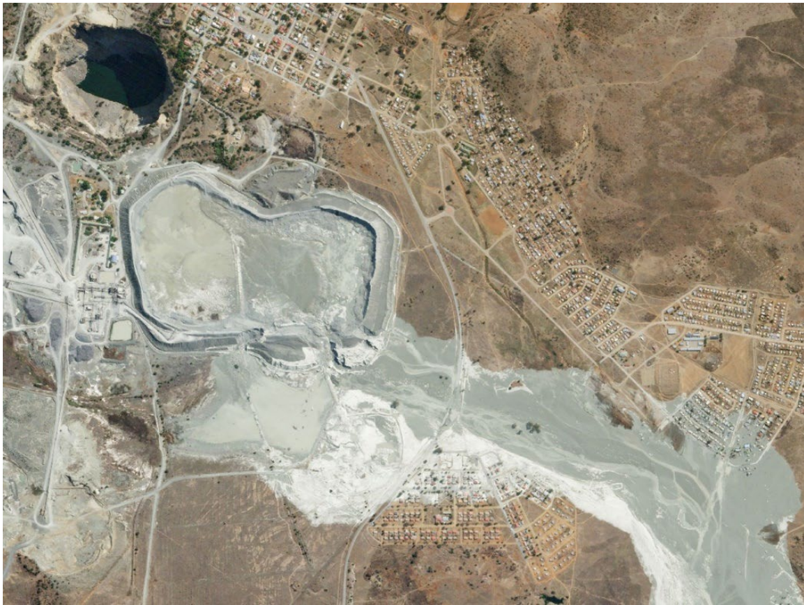
FIG 1 – Jagersfontein tailings dam failure, South Africa (Planet, 2022).
