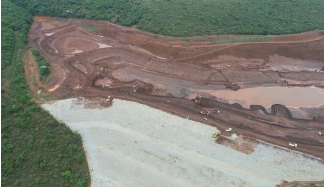
FIG 9 – Stage 3 mining operation.
