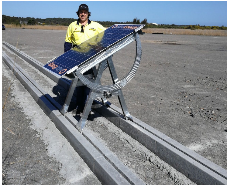
FIG 7 – Vales Point ash dam trial foundations.
