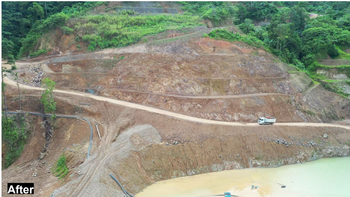
FIG 3 – Batter after stabilisation works..
