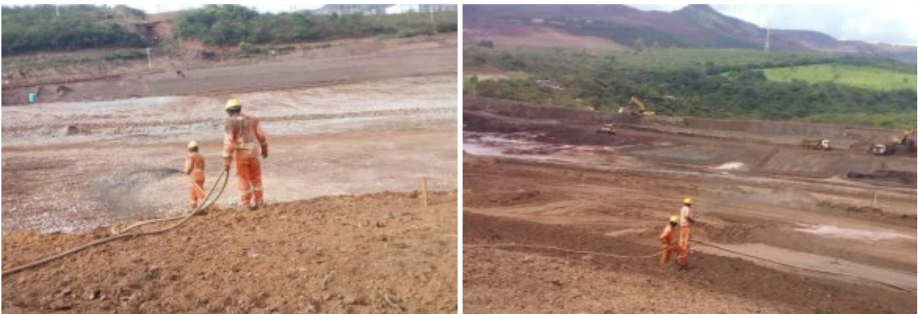
FIG 12 – Hydroseeding process.
