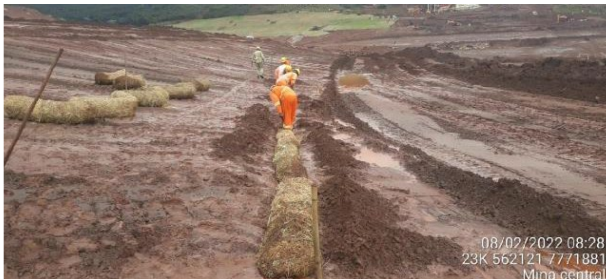
FIG 13 – Sediment retainers.
