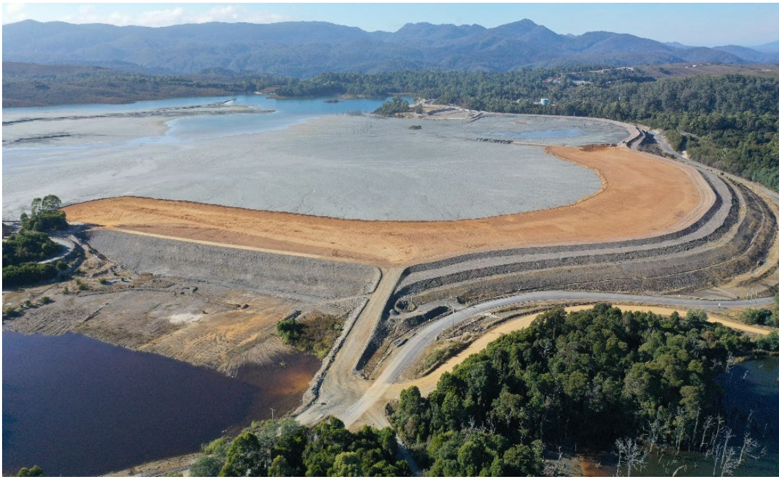
FIG 9 – Clay cover placement.
