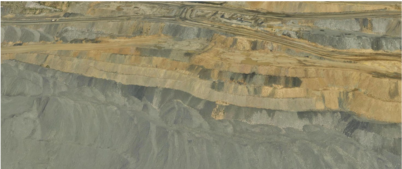
FIG 5 – Successful implementation of 10 m high lifts.
