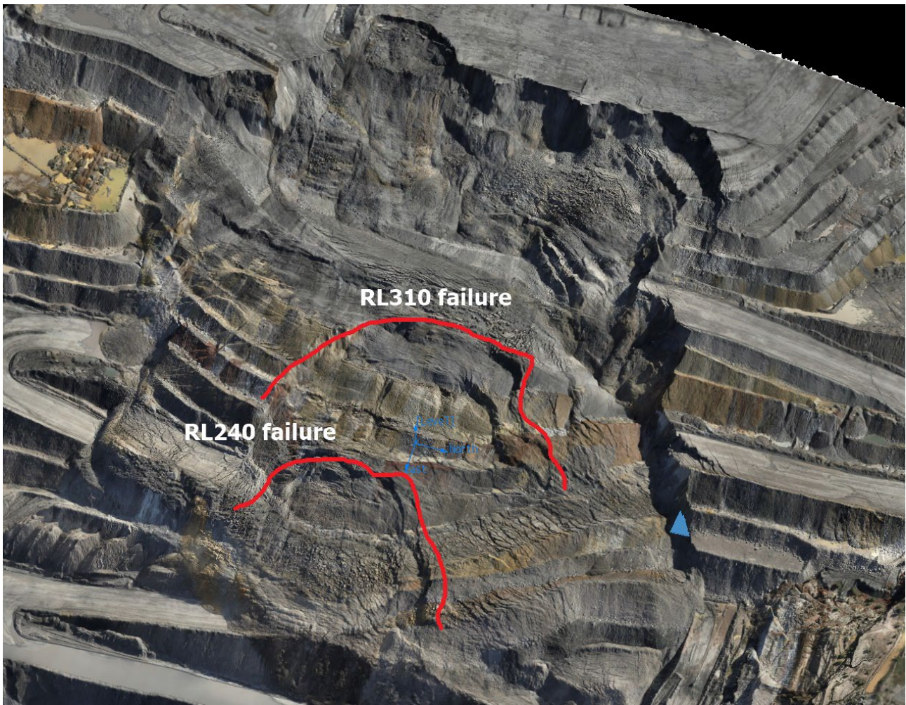
FIG 4 – UAV photogrammetry taken 4 July 2022, with initial instability at RL310 and subsequent instability at RL240 visible as back scarps within overall failure mass.
