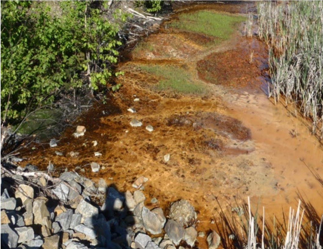
FIG 1 – Precipitation of ferric iron precipitates at the toe seepage point.
