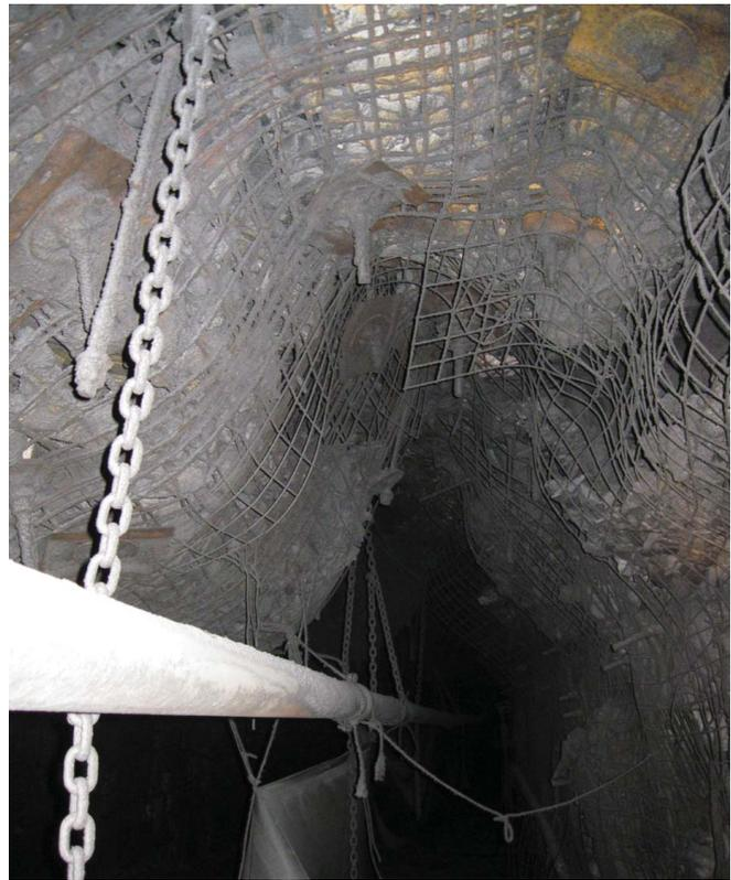
FIG 2 – ‘Guttering’ of roof (at the development face).
