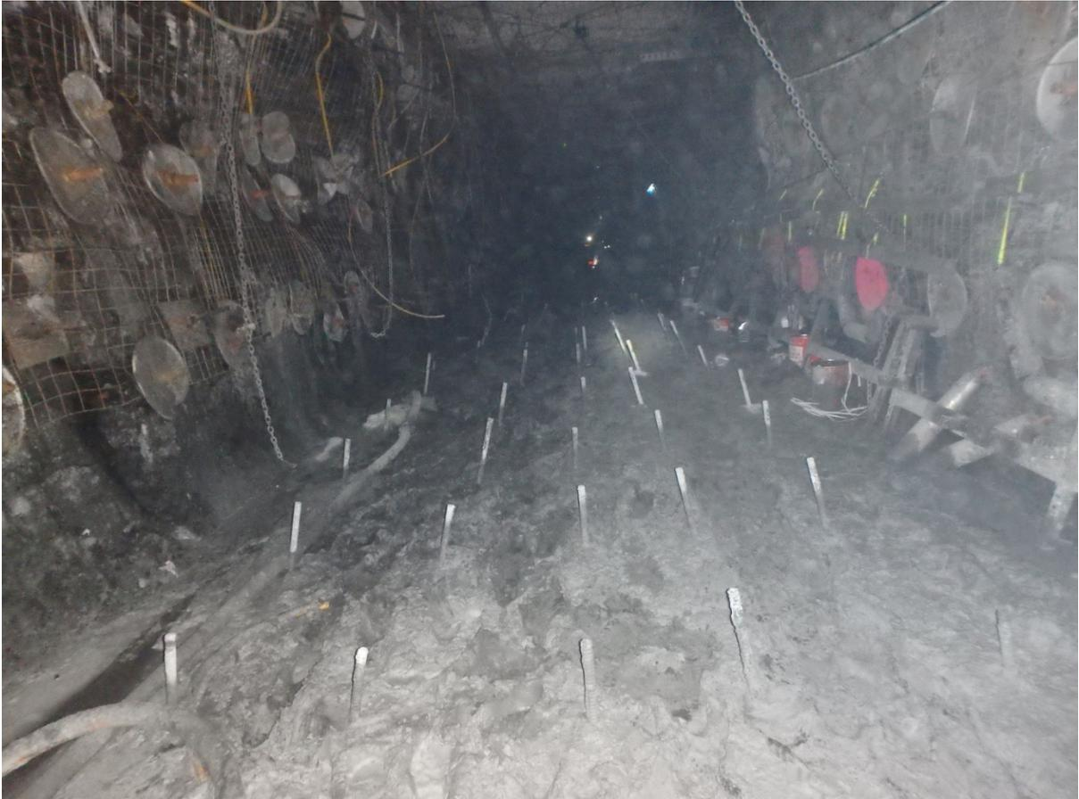
Figure 20 LW421 recovery area floor reinforcement
