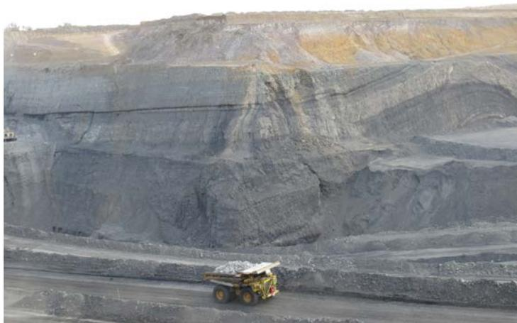
FIG 1 – Example of case study in which slope failure spanned multiple benches
