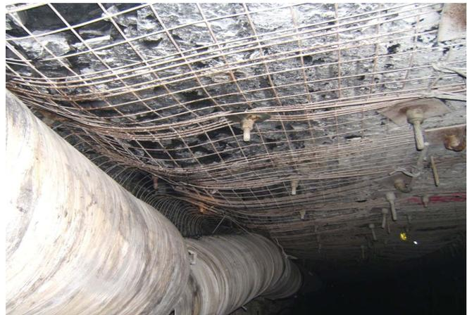
FIG 3 – Buckling of roof in outbye roadway (weeks post-development).
