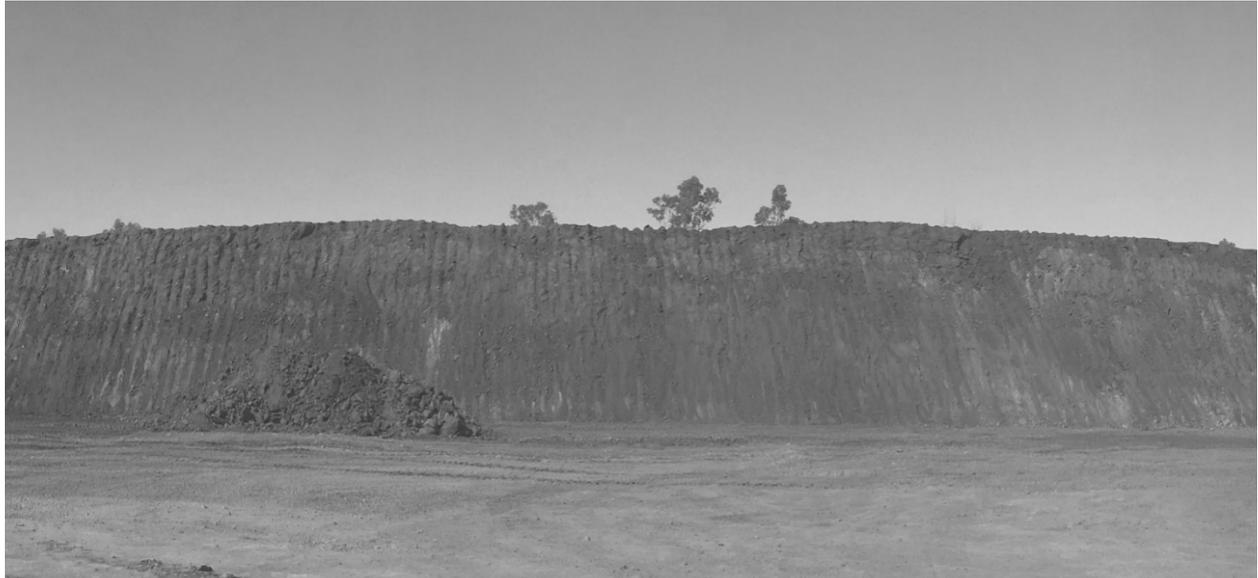
FIG 5 - Pit wall result using p-wave based timing and vibration modelling
