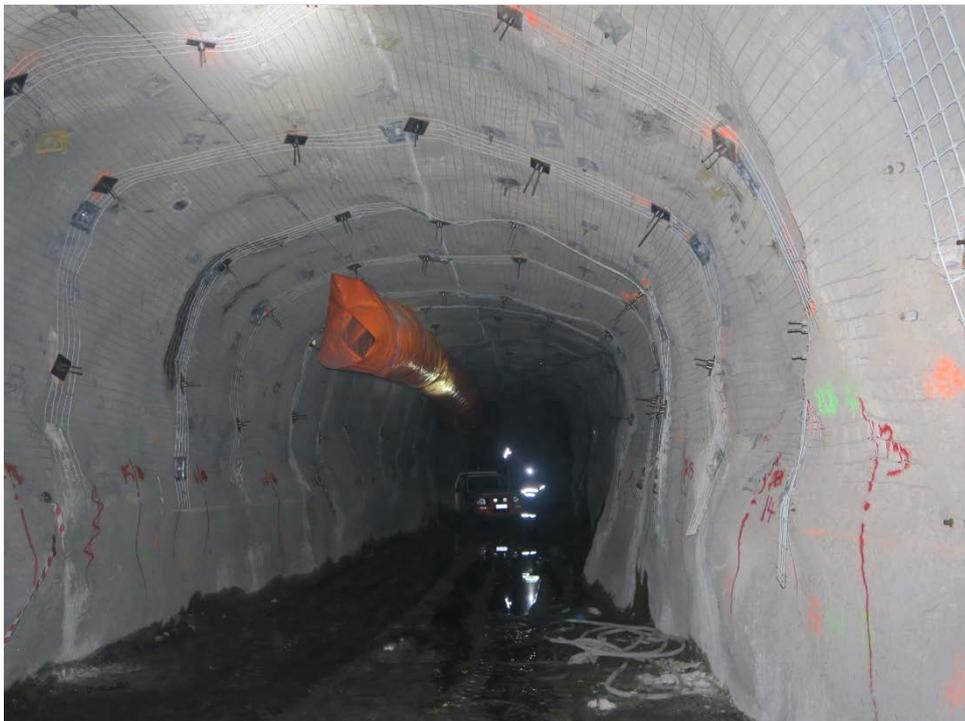
FIG 33: Improvements implemented: HS Profile, galvanised mesh, galvanised bolting and fibrecrete extended down to floor, twin-strand cablebolts, Osro straps (cables installed through the straps); mesh is installed over the fibrecrete.
