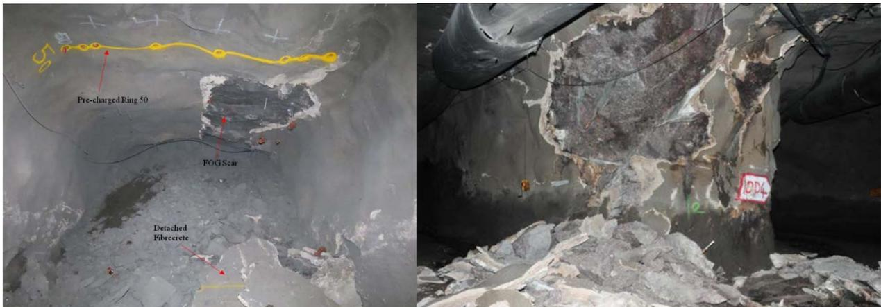
FIG 20 and 21: Rockfalls ahead of cave front, fibrecrete as only surface containment support
