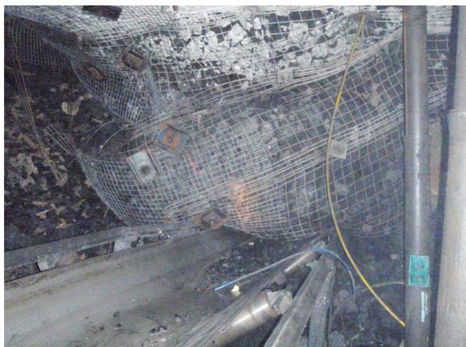
**FIG 4** – Roof fall on a belt road at Springvale (months post-development).
