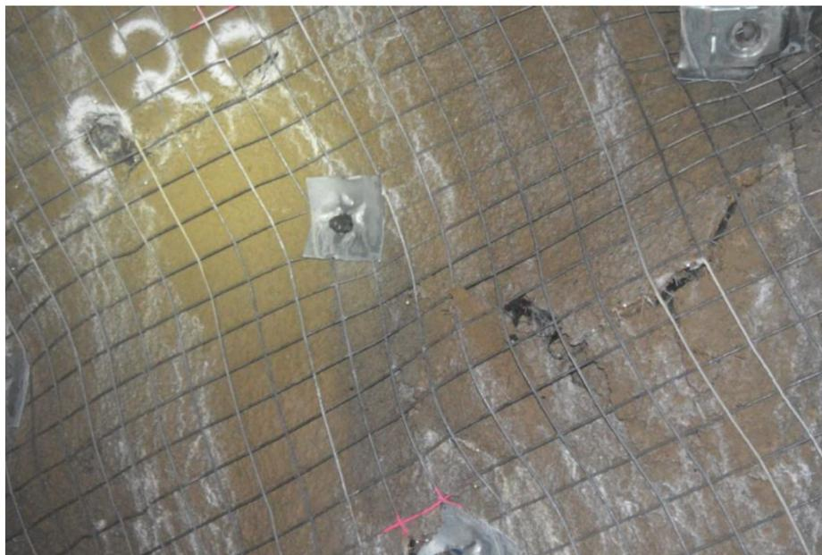
FIG 30: Resin rockbolts loaded, fibrecrete cracks due to rockmass dilation
