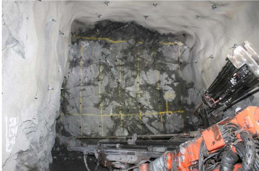
FIG 11: Fibrecrete and resin bolting square profile drive from early stages of EHM development
