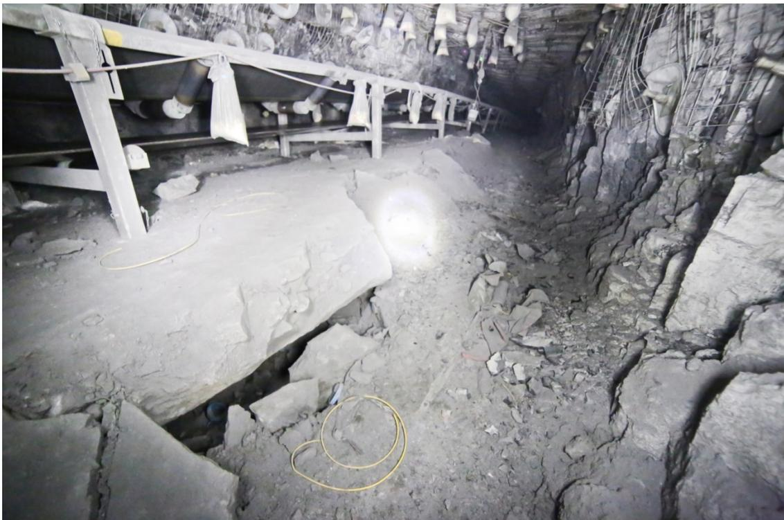
Figure 3 Floor Buckling at Springvale Mine
