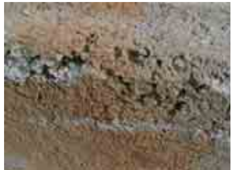
Photo of a poor concrete flow.
