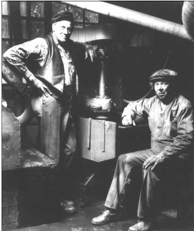
The first vertical pump, manufactured 1933.
