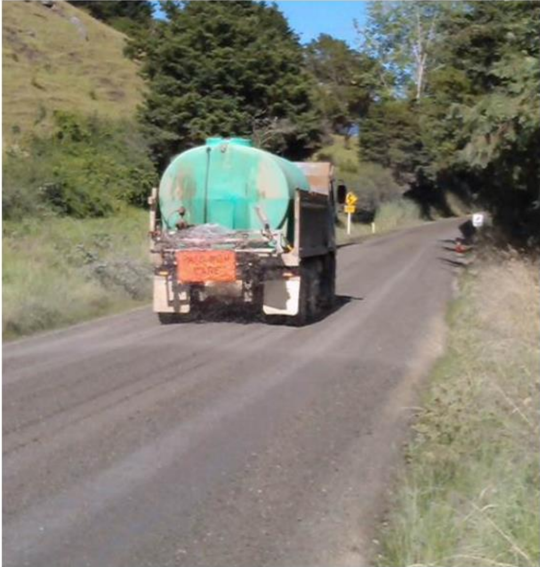
Figure 3.7 Application of magnesium chloride to Mataraua Road
